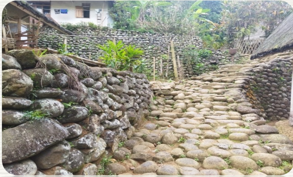
Arrangement of Erosion Resisting Stone ( Entep Stone )
